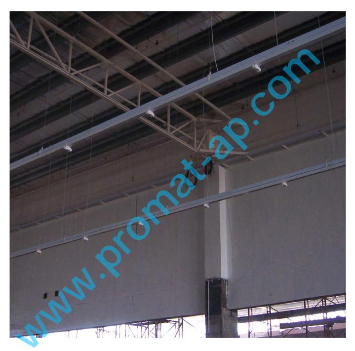
he purpose of a cavity barrier is to prevent the spread of smoke and flame from penetrating and/or moving within a concealed space in a fire compartment. Documents supporting the regulations provide guidance on where such barriers should be located within hidden voids in a building and they usually give examples of deemed-to-satisfy barriers for voids in stud walls or partitions.
